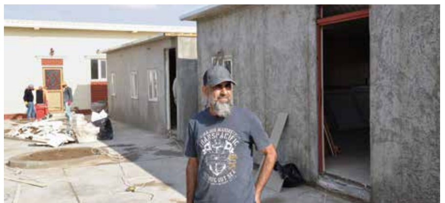
New construction in Bakhda.
