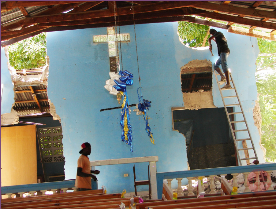
Repair of the church of Magagnosse in Haiti after it was heavily damaged by Hurricane Matthew in 2016.
