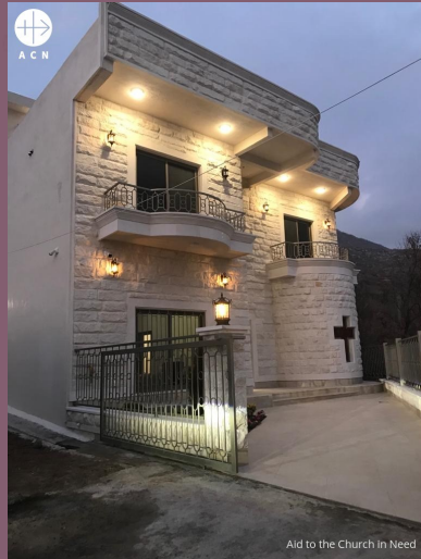
The new centre for the Sisters in Araden, northern Iraq.
